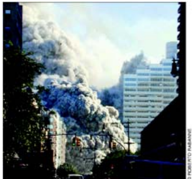
Fig. 1.1.2 The overall collapse of WTC7
