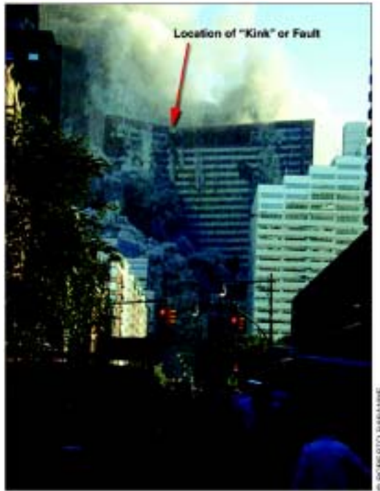
Fig. 1.1.1 view from the north of the “kink” or fault developing in WTC7
