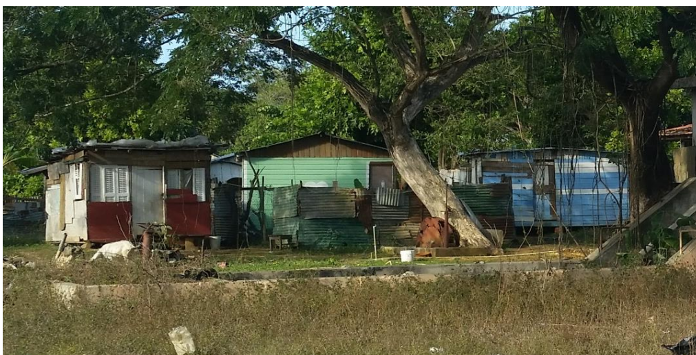
Figure 2-4 Typical Timber Houses in a Squatter Settlement or Informal Settlement in Jamaica. Source: Fieldwork 2017
