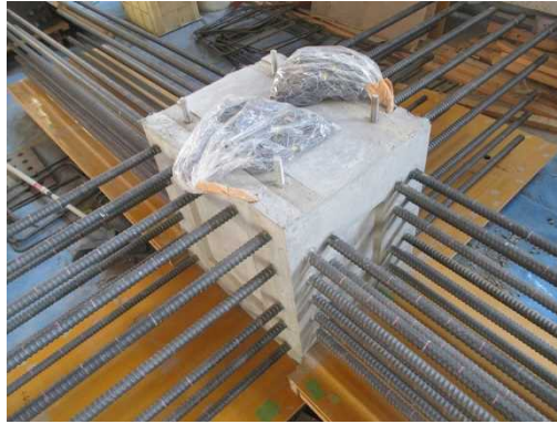
Fig. 3. 7 Demolding
