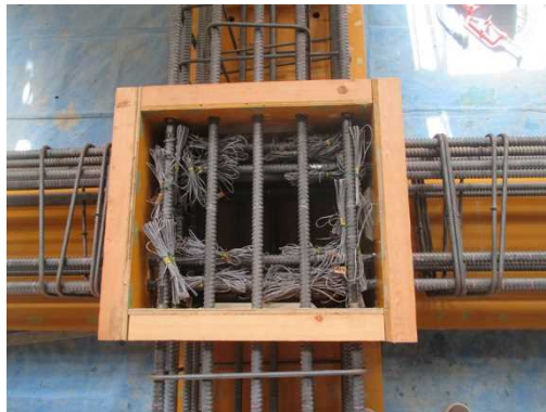
Fig. 3. 5 Mold for panel zone
