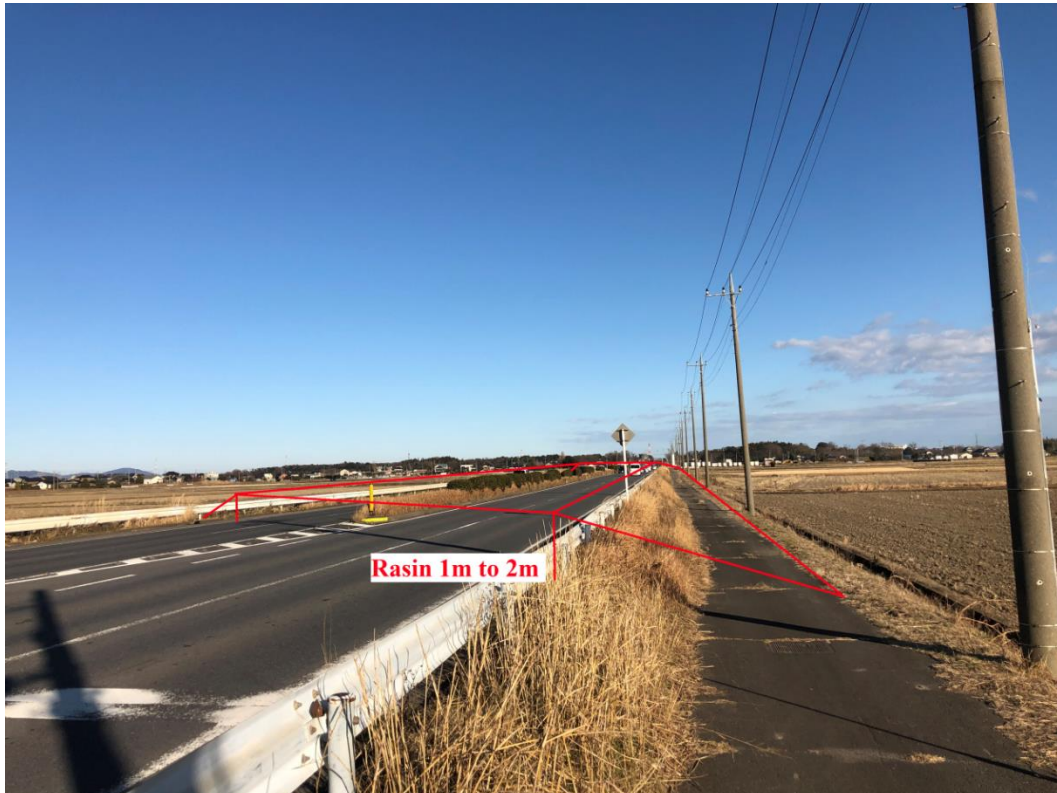
Figure 5-29 Image of the raised road by 1 to 2 meters
