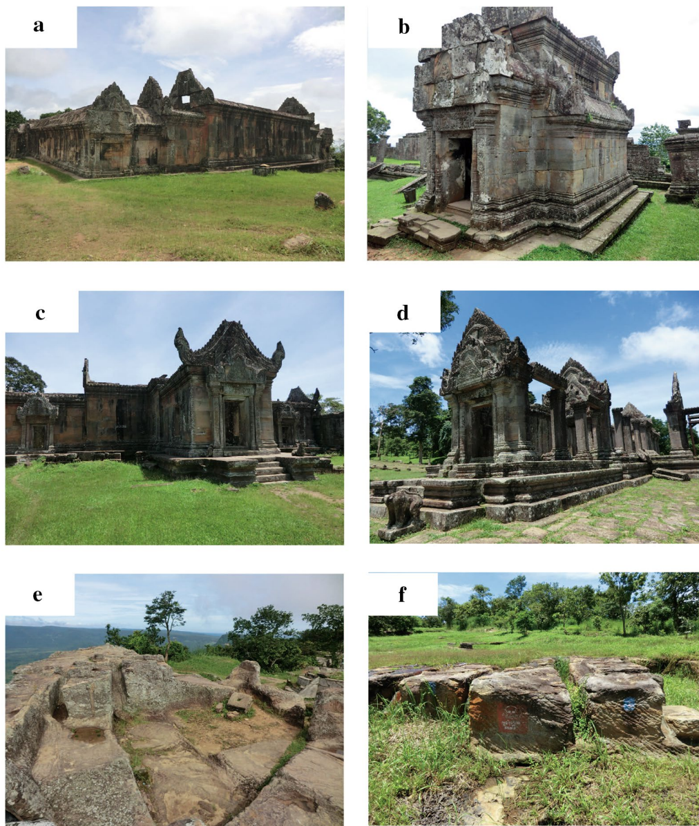
Fig. 3 Photographs of (a) South Gopura (A) and Gallery (D), (b) Eastern Library (H1), (c) Gopura III (P), (d) Gopura IV (T), (e) ancient sandstone quarry for large sandstone blocks situated in the south of South Gopura (A), and (f) ancient sandstone quarry situated in the west of the causeway between Gopura IV (T) and Gopura V (W). Sandstone blocks used for these building have a yellowish-brown color
