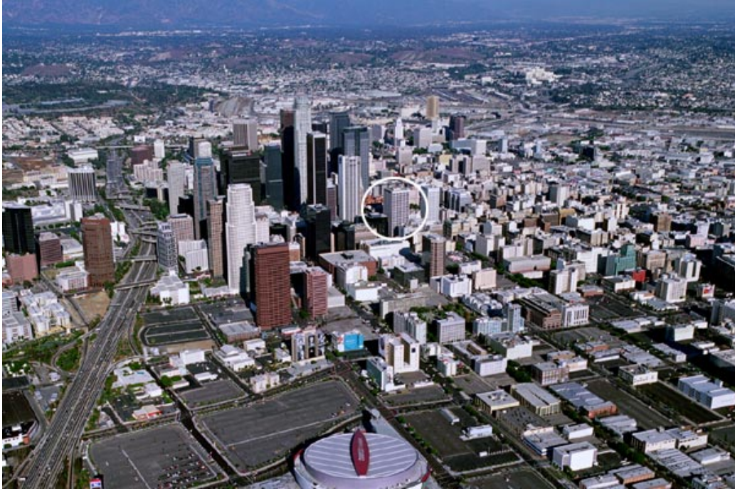
Figure 6.1: One Wilshire in Los Angeles houses one of the largest groupings of datacenters in the world
