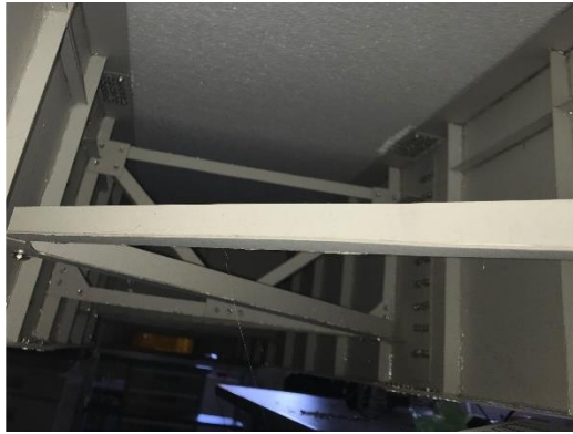
(c) Lateral bracing
