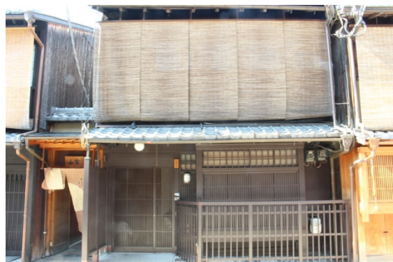
d: wooden buildings
