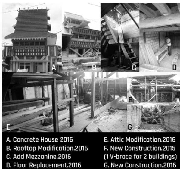
Figure 7 New Construction and modification in Omo Hada.
