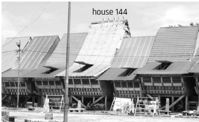
Figure 9 House number 144 in raya area. Source : Author
