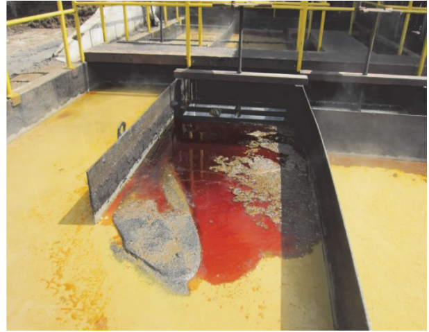
Fig. 3. Oil-containing wastewater generated at a palm oil factory in Thailand.
