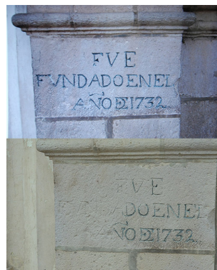
Figure 31: Cleaning the Los Dolores church led to damage to one of its inscriptions (pictures show before and after cleaning). Interventions are regulated by law, but little knowledge of the Heritage Law, which applies to all government workers, allows such damage to happen. Source of the image: http://www.latribuna.hn/2015/07/13/danos-irreversibles-a-iglesia-los-dolores/
