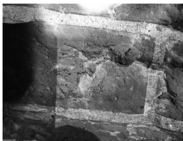
Figure 2: Salt weathering
