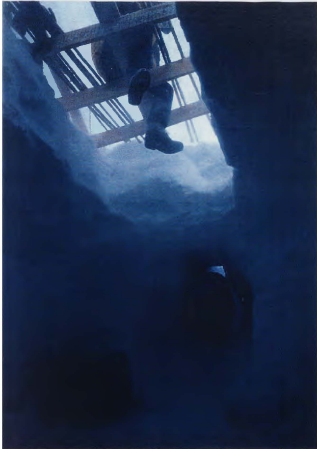
Figure 8. Roof of the drilling trench. The roof was made by wood and bamboo poles and covered with plastic canvas.
