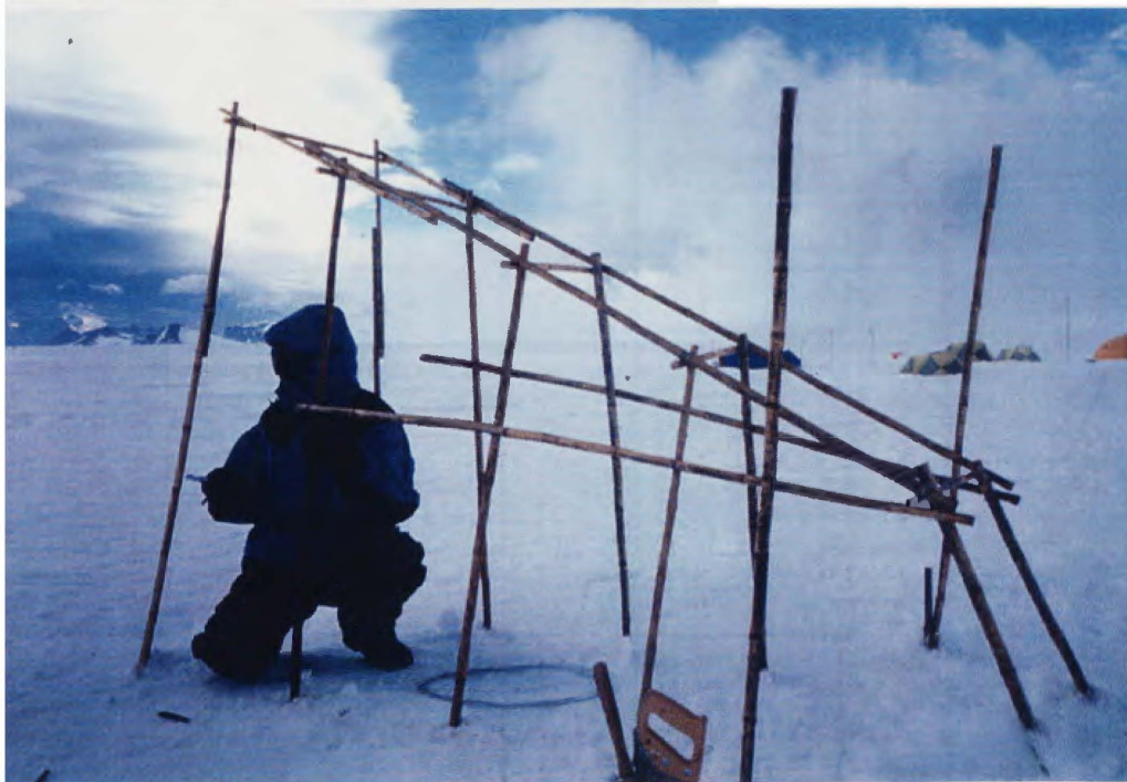
Figure 9. Entrance of the drilling trench. The bamboo structure was later covered with plastic canvas.
