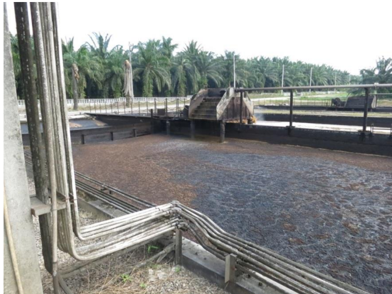
Fig. 1.8 Open pond for methane fermentation using wastewater from the palm oil factory
