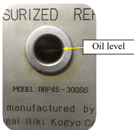
(1) Oil level for gearbox
