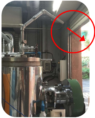
(6) Steam leak pipe on top of the pressurized hopper
