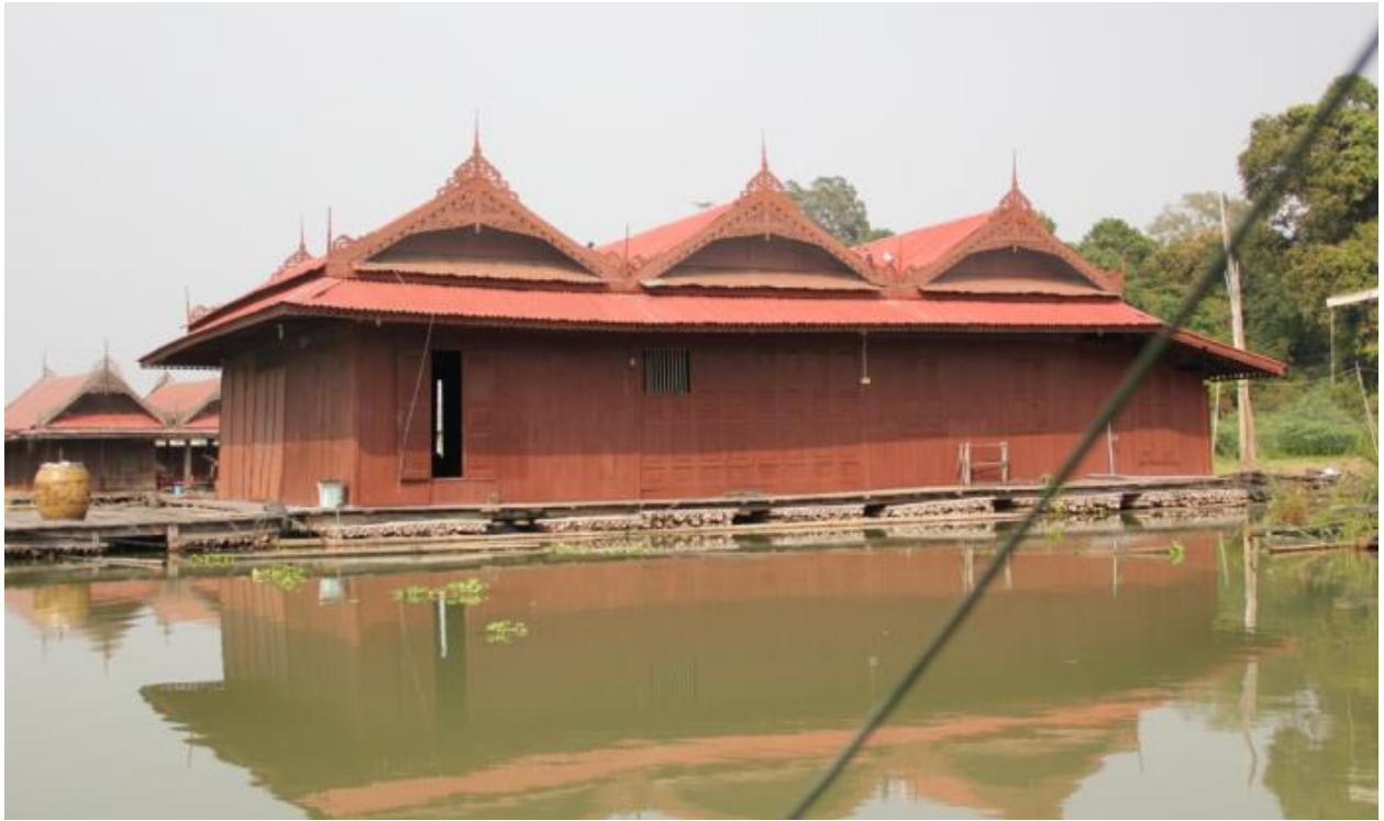
Figure 113 Raft house No.1 in Sakraekrang River community
