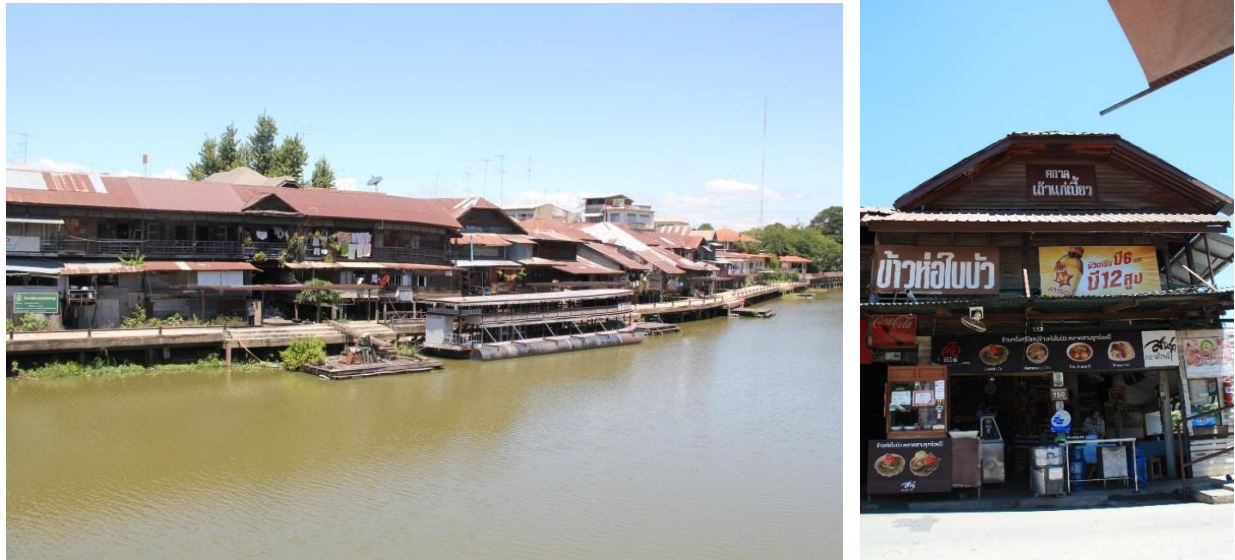
Figure 95 Associated structure No.2 (of Taokea Baeu's market building) in Talad Samchuk community
