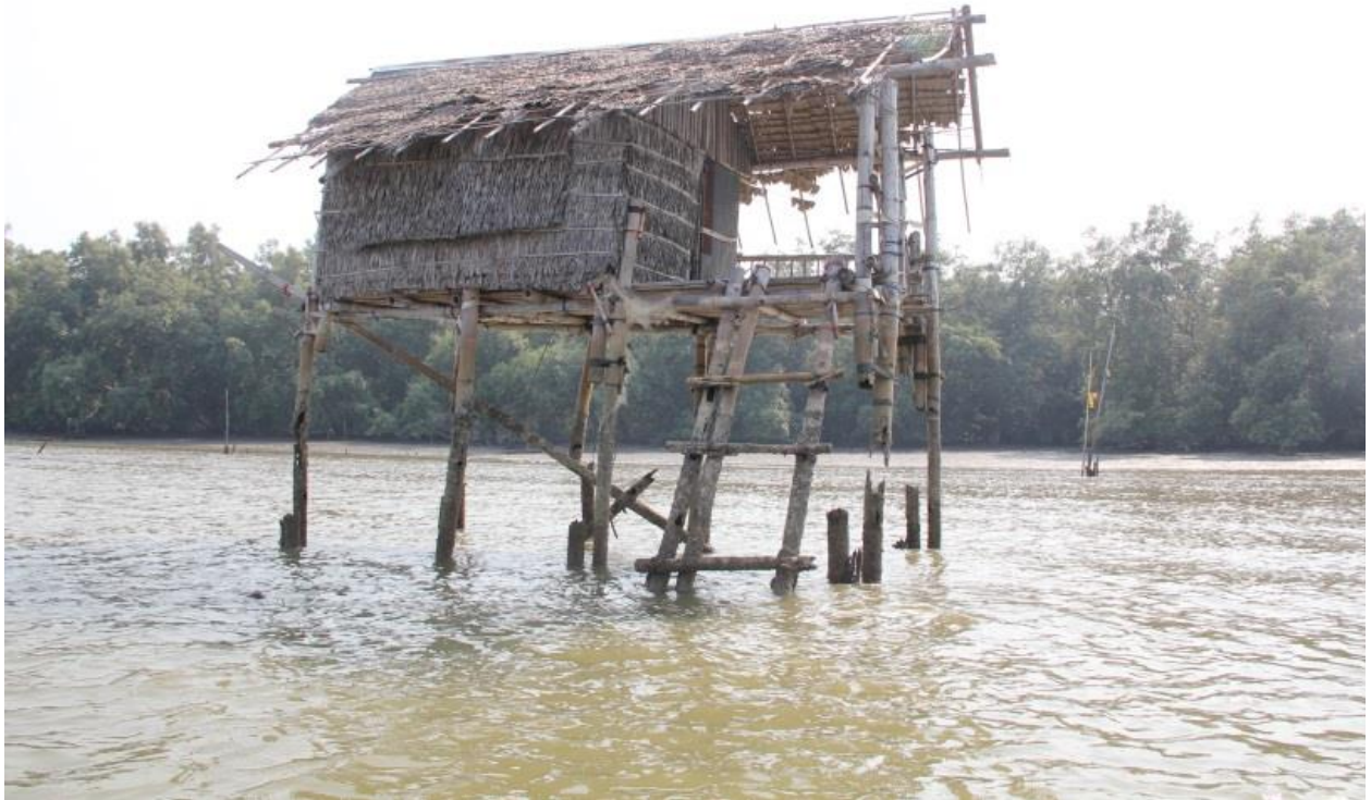
Figure 85 Associated structure (offshore shelter) in Leamyai community
