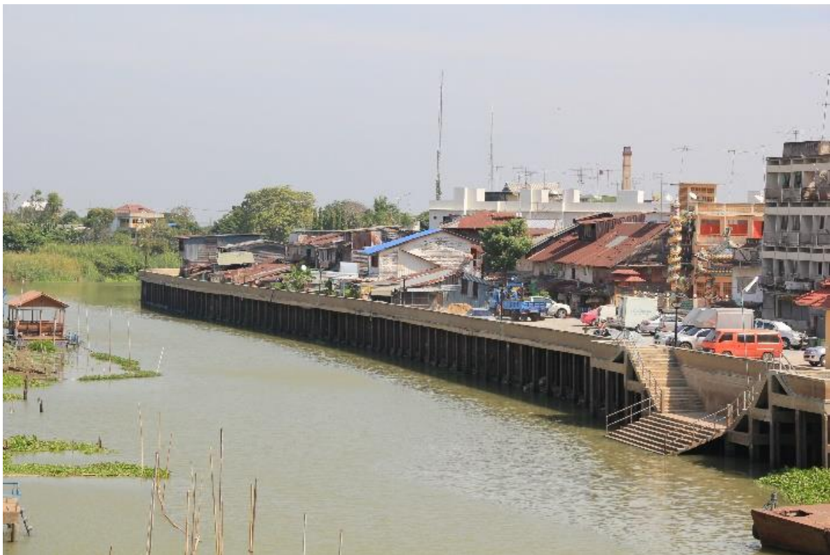
Figure 100 New waterfront structure and flood barrier (which was at 5.5 meters height in some area)
