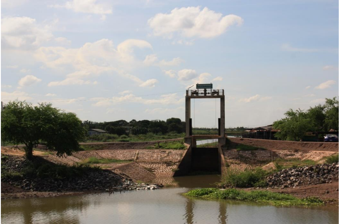
Figure 58 Water gates were constructed on existing rivers to control water flow in the dry season.
