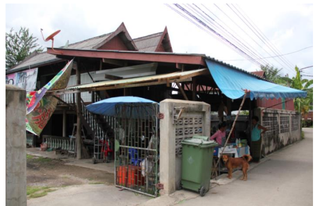
Figure 71 Traditional house no.2 in Yeesarn community
