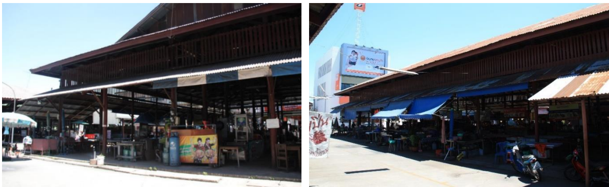
Figure 94 Associated structure No.1 (market building) in Talad Samchuk community
