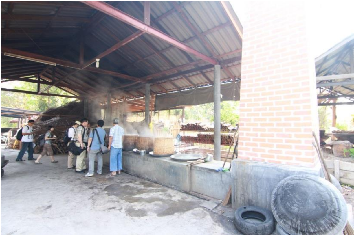
Figure 66 Associated structure no.4 (coconut sugar stewing plant) in Amphawa community
