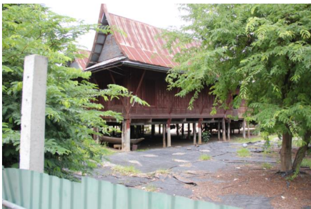
Figure 70 Traditional house no.1 in Yeesarn community
