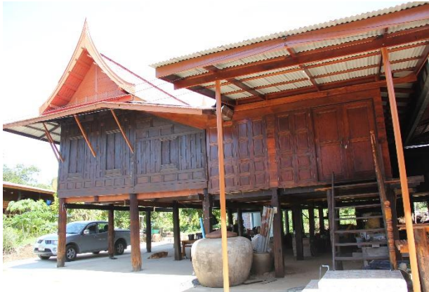
Figure 51 Traditional house no.3 in Pakkran
