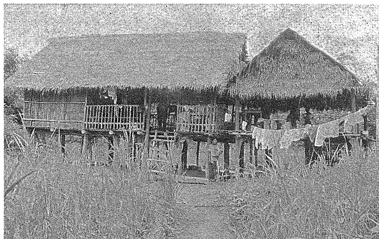
Fig. 6. Ribereño shelter. Homes are built of locally-available construction materials. Huacapú ( Vouacapoua americana ), resistant to rot, is used as main posts, while palm trunks and fronds are employed for thatching and flooring. Floors are raised between 1.0–2.5 meters above the ground for protection from floods and for comfort.
