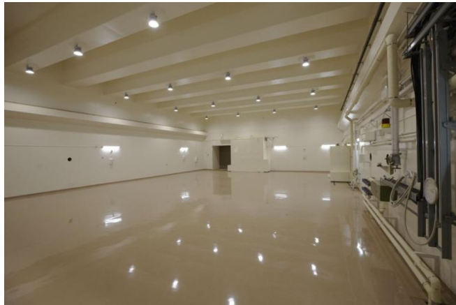
Figure 1. Photograph of the accelerator room after the completion of renovation work.
