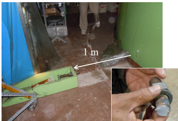
Fig.12 Photo of the moved shock prevention devices at the 7th floor.
