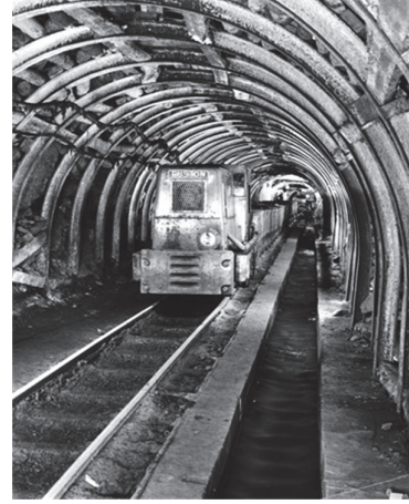
FIGURE 2: The haulage roadway.
