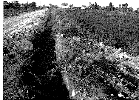
Figure4 Slim flow of canal in Minqin
