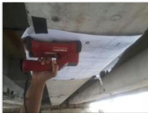
Figure 5-10 Concrete cover assessment
