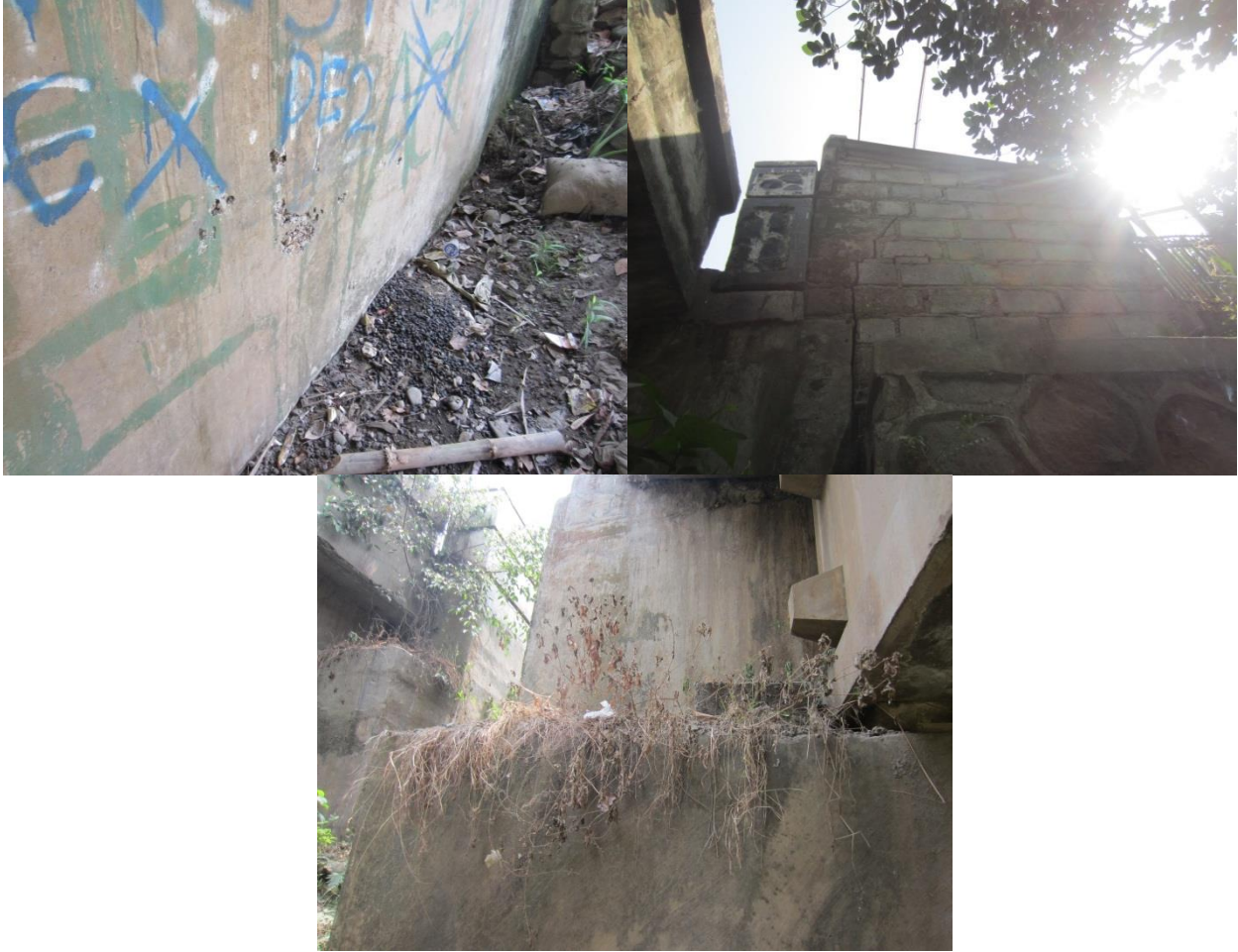
Figure B.7 Abutment
