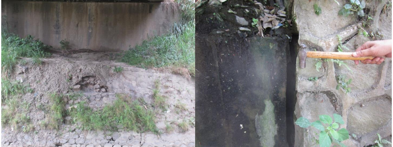
Figure B.5 Scour Protection
