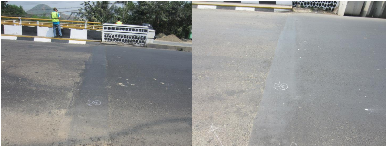
Figure B.11 Deck joint
