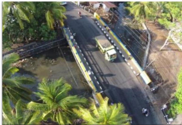
Figure 5-7 Matani Bridge bird view
