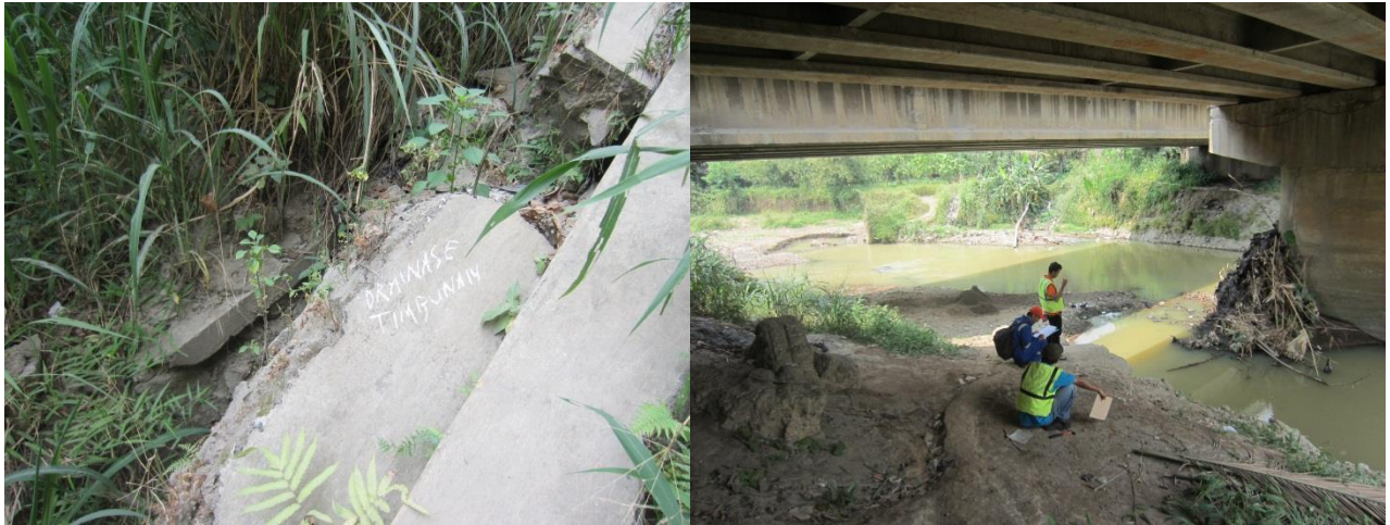
Figure B.6 Embankment and channel
