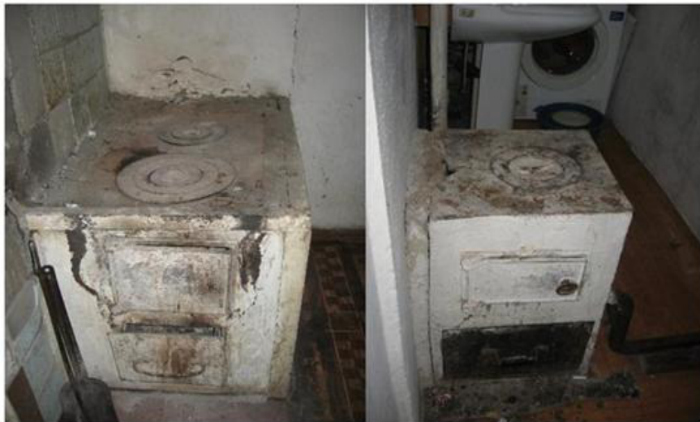
Figure 5.28 Typical home-made coal stoves used for space heating in rural areas of Kazakhstan without centralized heating system
