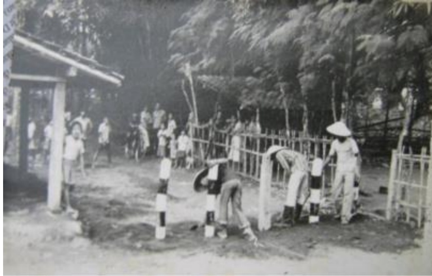
Figure 22. Concrete blockages setting (source: Sucoro)
