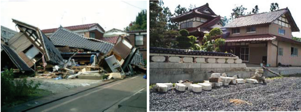
Fig. 1. Comparison of the lightly damaged house, which was built in 1980, Iwate-Miyagi inland earthquake, 2008 ( M_j 7.2), Ishinomaki, Miyagi prefecture (left: photo. by T. Ohsumi photo taken on 15 June, 2008) and the collapsed house in Niigata Chuetsu-Oki earthquake, 2004 ( M_j 6.8), Kawaguchi, Nigata, prefecture, (right: photo. by T. Ohsumi taken on Oct.,2004).
