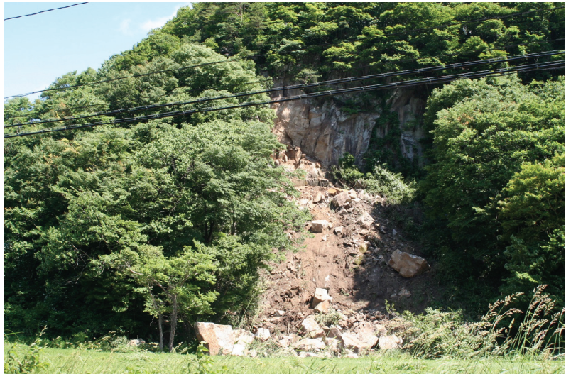
Fig. 19. Full view of Ichinoseki Genbi-Itagawa small-scale slope collapses near National Route 342.
