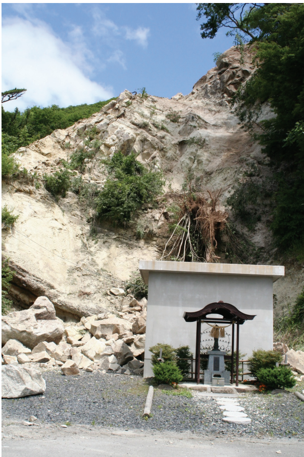
Fig. 24. Full view of downstream left bank occurred the middle-scale collapses.
