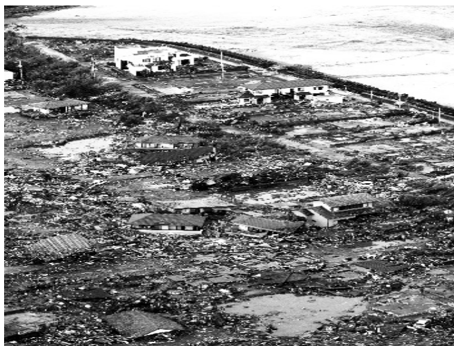
Figure 4 Kita Ibaraki Seaside Damage from 3-11 Tsunami (Photo: Asahi Shinbun)
