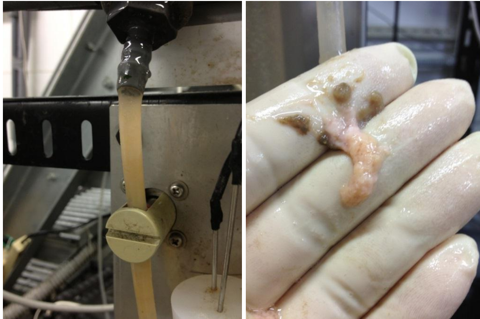
Picture 2-12 Deposits removed from influent tube during maintenance
