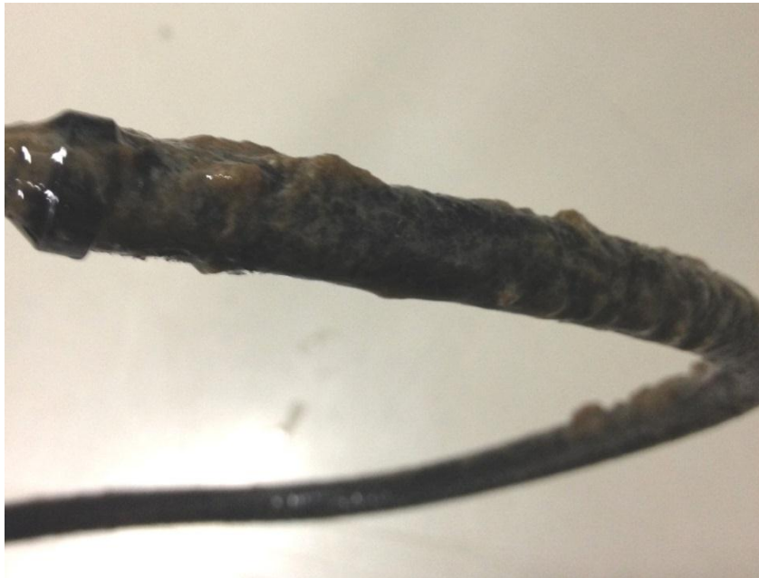
Picture 2-9 Diffuser fouled by slime, filaments and worms.
