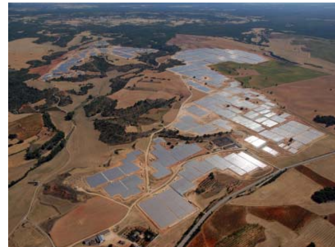
Parque Fotovoltaico, Olmedilla de Alarcon, Spain 60MW, Constructed September 2008
