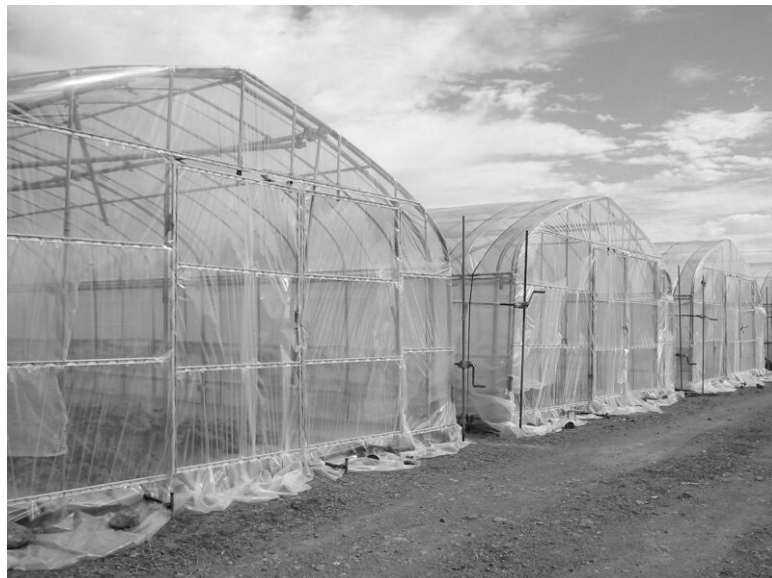
Fig. 5.1 Common two or more single-span pipe houses stand in a row in the field.
