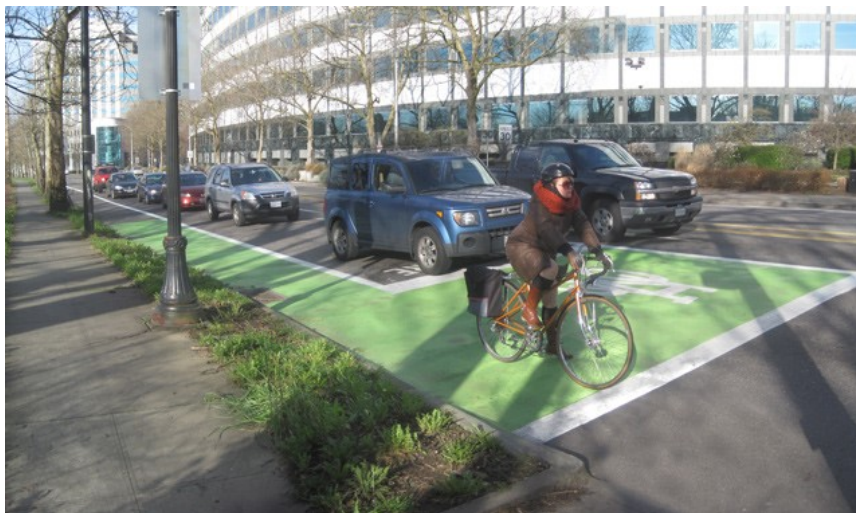
Figure 1-15 A bike box in Portland, USA
