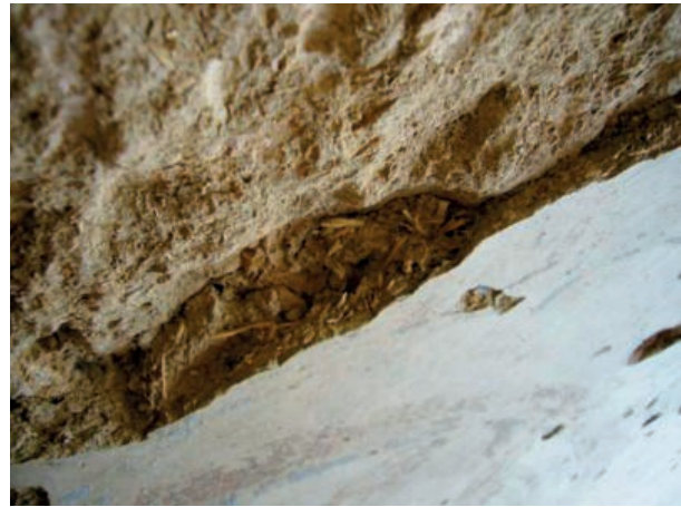
Figure 2.4 A layer comprised of fine fibres, possibly from cow dung, between the rock surface and the earthen render (Cave I, niche). Photo: Y. Taniguchi, courtesy of NRICPT, 2006.
