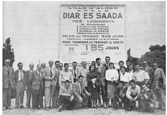
FIGURE 8. Pouillon's team at a building site ( Algiers Revue 1954–3)
