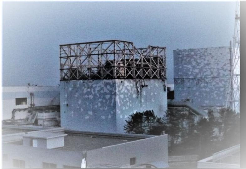
**Fig. 1.** Damaged Unit-1 reactor of Fukushima Daiichi, viewed from the north-west side. The Unit-2 building is seen to the right. (Courtesy of TEPCO, the Tokyo Electric Power Company Ltd.)
