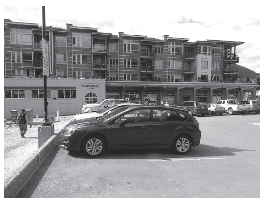
Fig. 13 Store and apartment complex of the Kootenay Co-op
