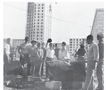
Fig.6 Party for construction laborer in Diar es-Saada (Alger Revue 1954-8)
