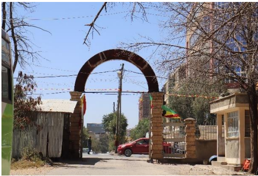
Figure 4-8 Tigrai Court Building originally built for Italian administration office. By author.
