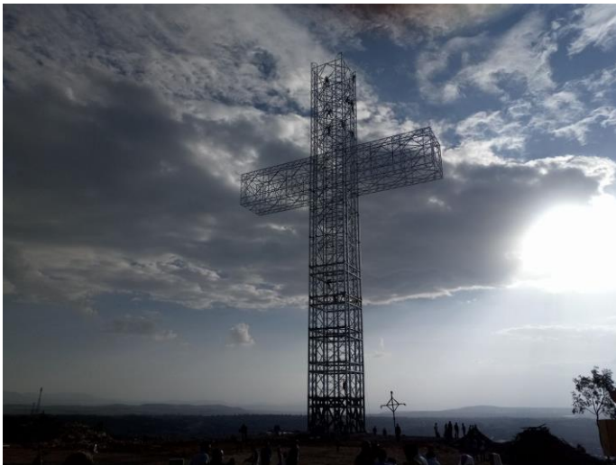
Figure 5-29 A Picture of 52 meter cross erected at the mount Chomea 168
