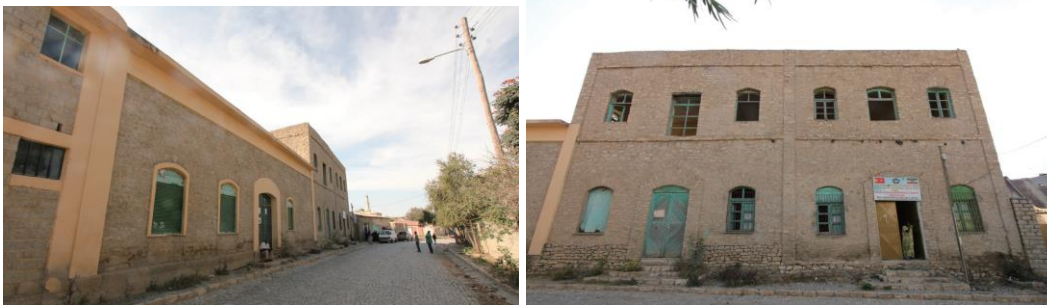
Figure 5-34 External appearances of Liquor factory building. Figure 5-35 Front view of Liquor factory building. By Shimizu, N. 2016
