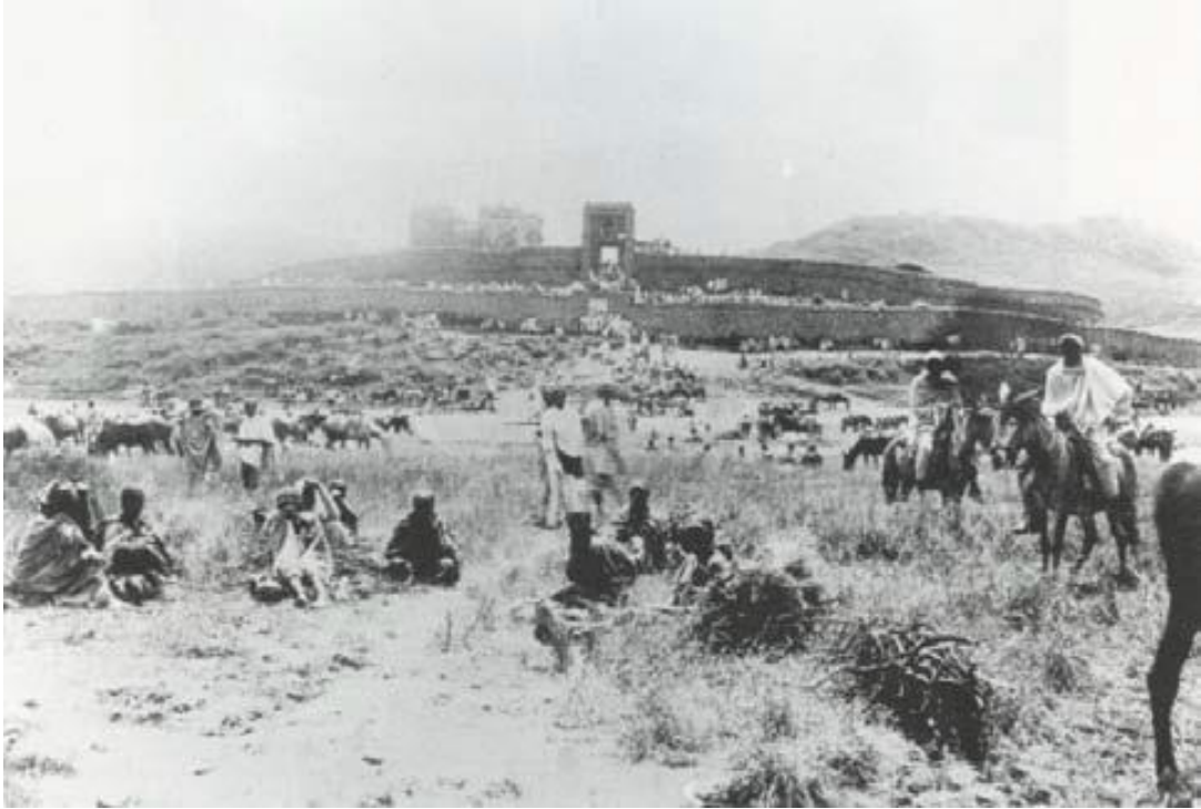
Figure 5-3 People in Market activity in front of Yohannes IV palace compound. 154
