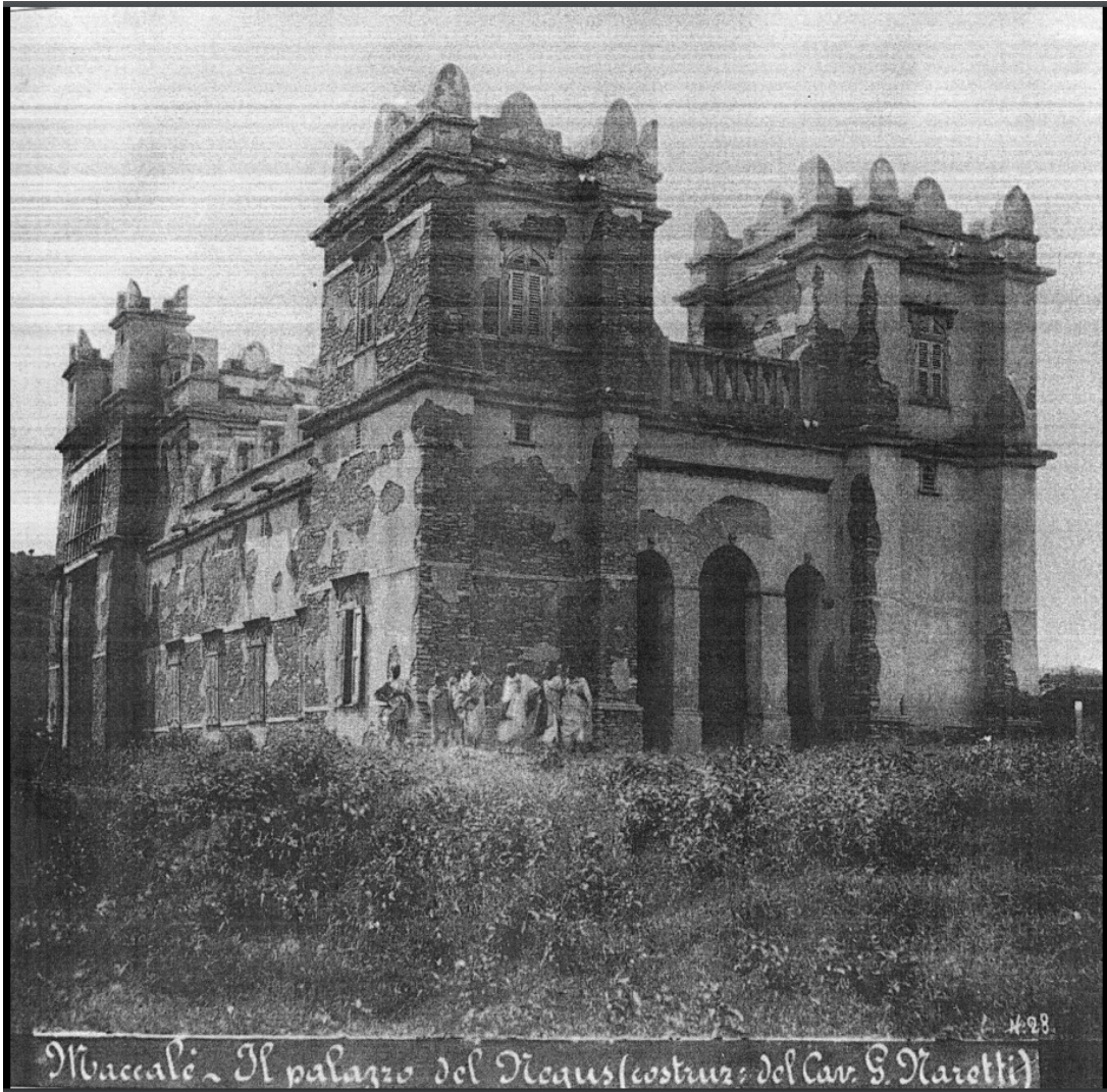
Figure 5-5 Deteriorated building Yohannes IV palace with falling plasters. Date unknown 156
