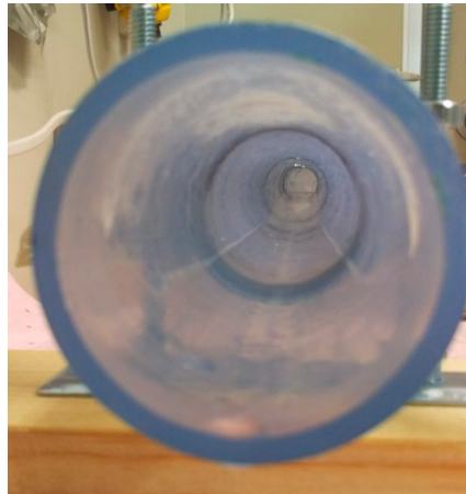
Figure 6. Sewer pipe blockage condition on the 7th day from the simulated experiment (Observation point 4).
