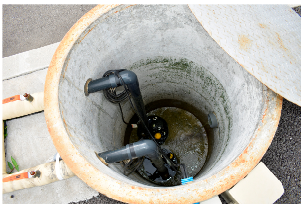
Figure 4. Pumps for harvest in cultivation sub-unit at Minamisoma ( 0.55 \text{ kW} \times 2 \text{ units} ).
