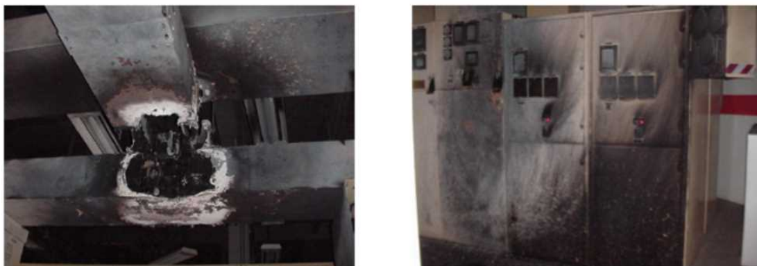
Fig. 2.2-4 Photographs of the HEAF event at Diablo Canyon NPP [10]
