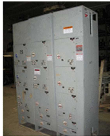
Exterior of MCC
