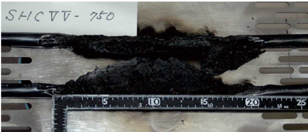
SHCVV cable temperature 550°C
