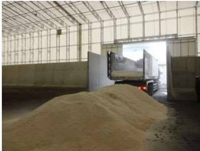
Fig. 6.1-1 Receiving equipment for waste gypsum board in Kyusyu plant.
