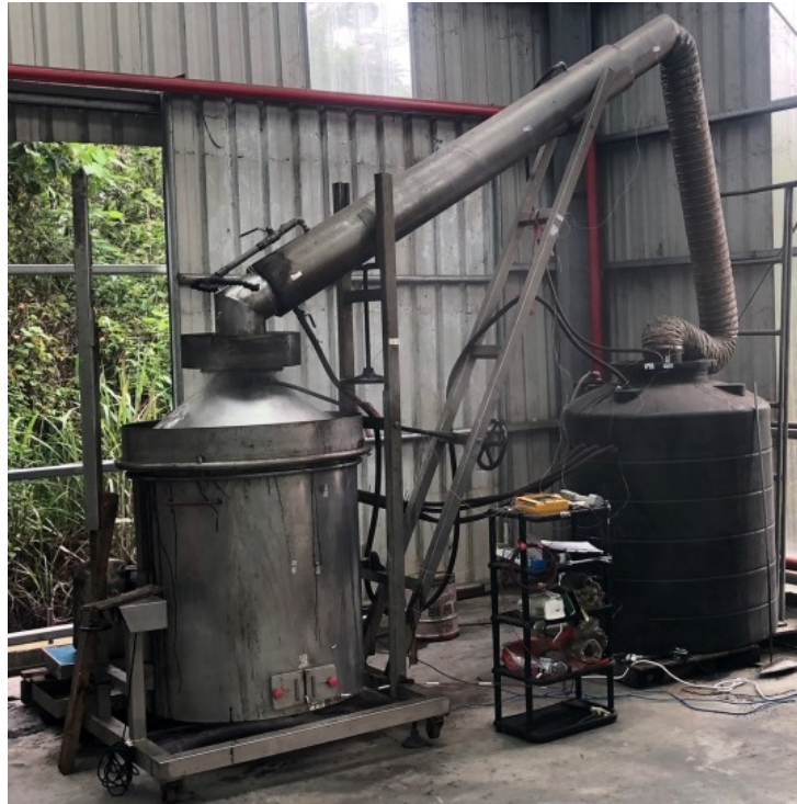
Fig. 2-5c Operation photos of CPSICF
