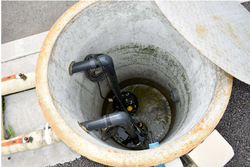
Fig. 1-4 Pumps for harvest in cultivation sub-unit at Minamisoma (0.55 kW × 2 units)
