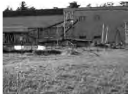
Fig.1 Surrounding condition near the trench at TERC covered with turf
