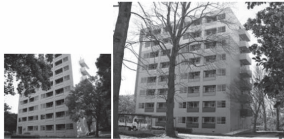
Before Refurbishment After Refurbishment
