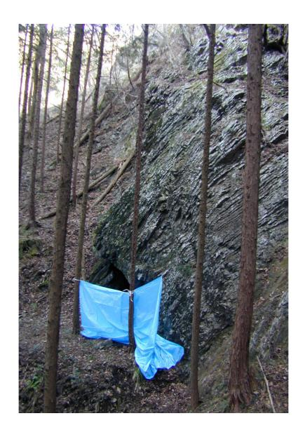
Photo 9: A rockfall trap at R-1 site in C3 watershed
